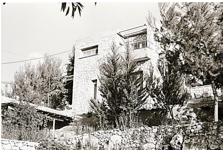
The house in Ramat Motza.
